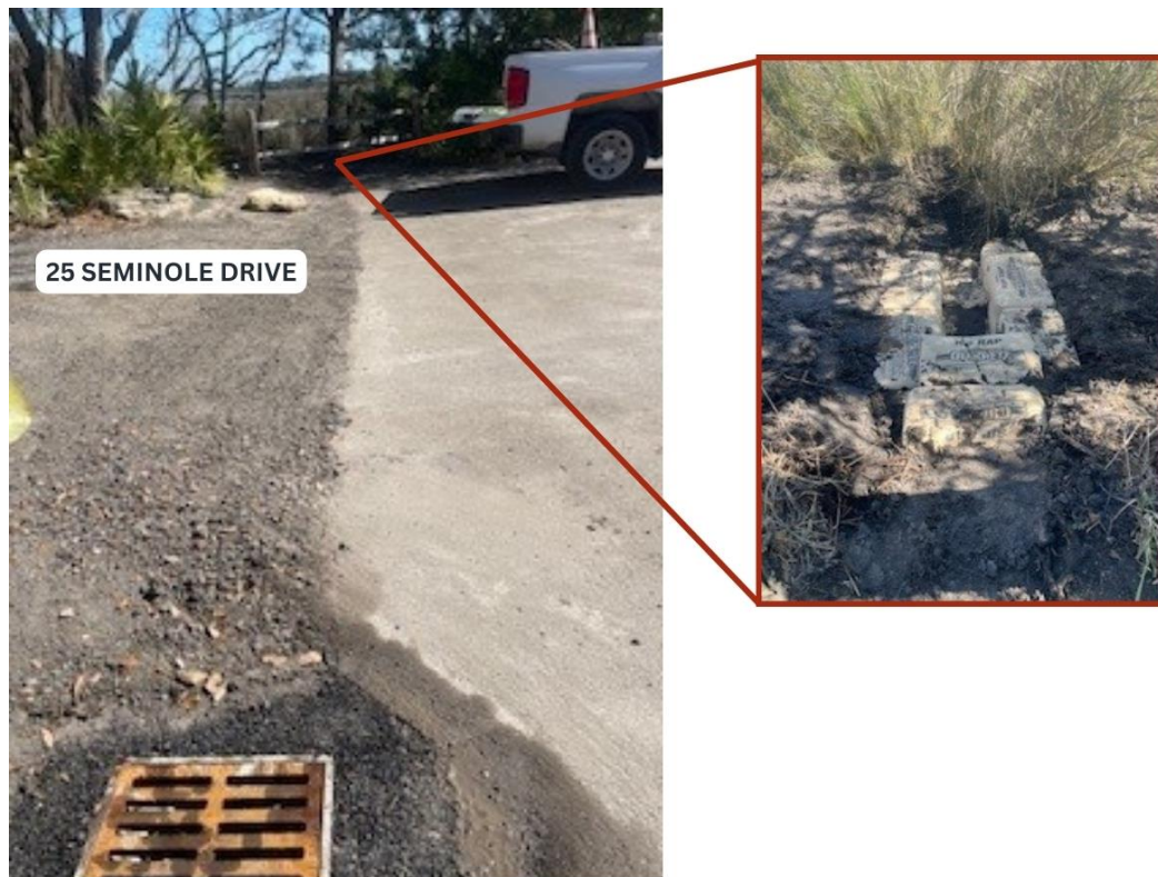
Figure 2-6 Newly Installed Inlet, Conveyance Pipe, and Outfall at Seminole Drive
