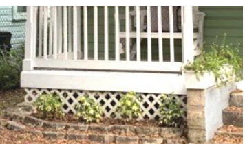
Example of Raised Pier construction with porous skirting (lattice). Image from ML+H.
