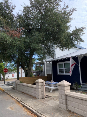
Masonry site walls with floodgates can provide flood protection. Image from ML+H.
