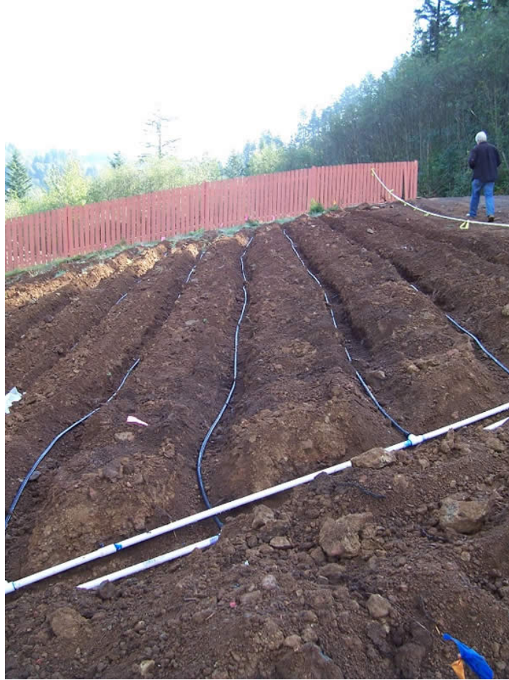
Figure 3-9 Example of a drip distribution system.
