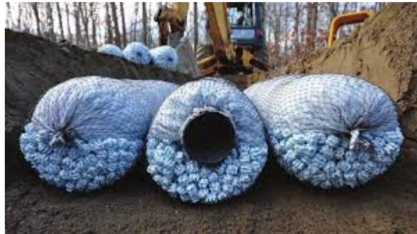
Figure 3-6 Example of an engineered aggregate unit.
