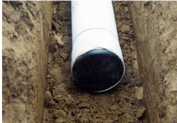
Figure 3-8 Example of a fabric-wrapped pipe.
