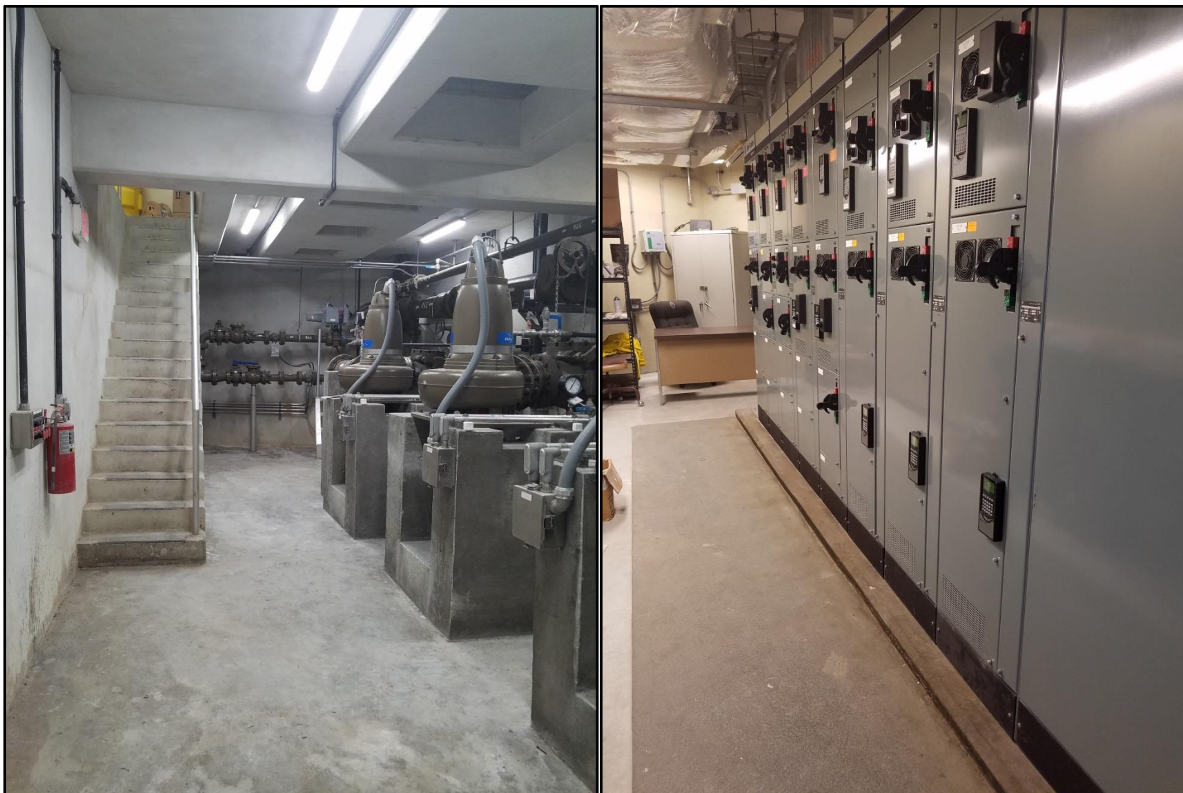
Figure 3: Photos of Existing RAS Pump Station Pump Room (left), MCCs in RAS Pump Station Main Floor (right)
