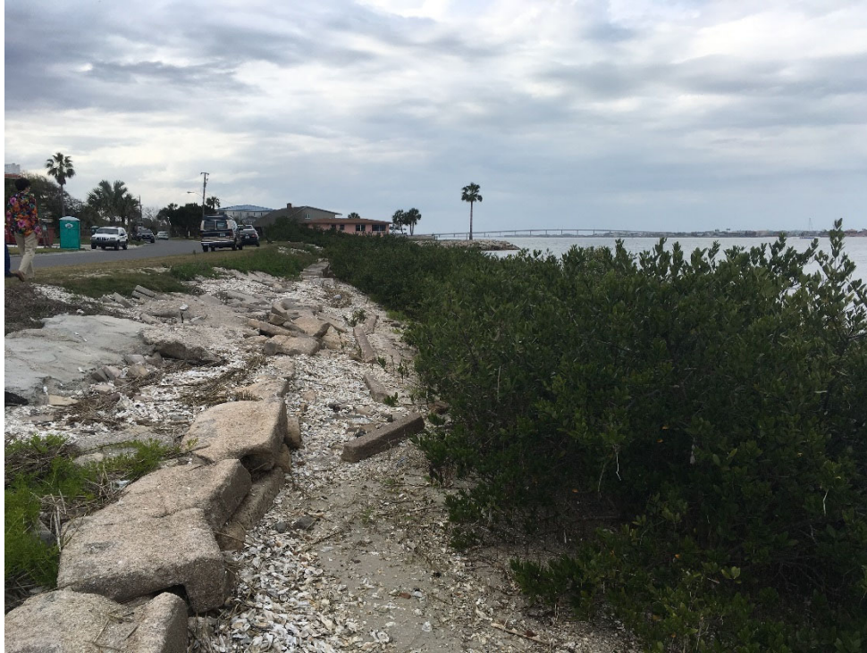
Figure 1. Remnant shoreline stabilization showing varied materials, crest elevations, and deterioration, as well as presence of mangroves
