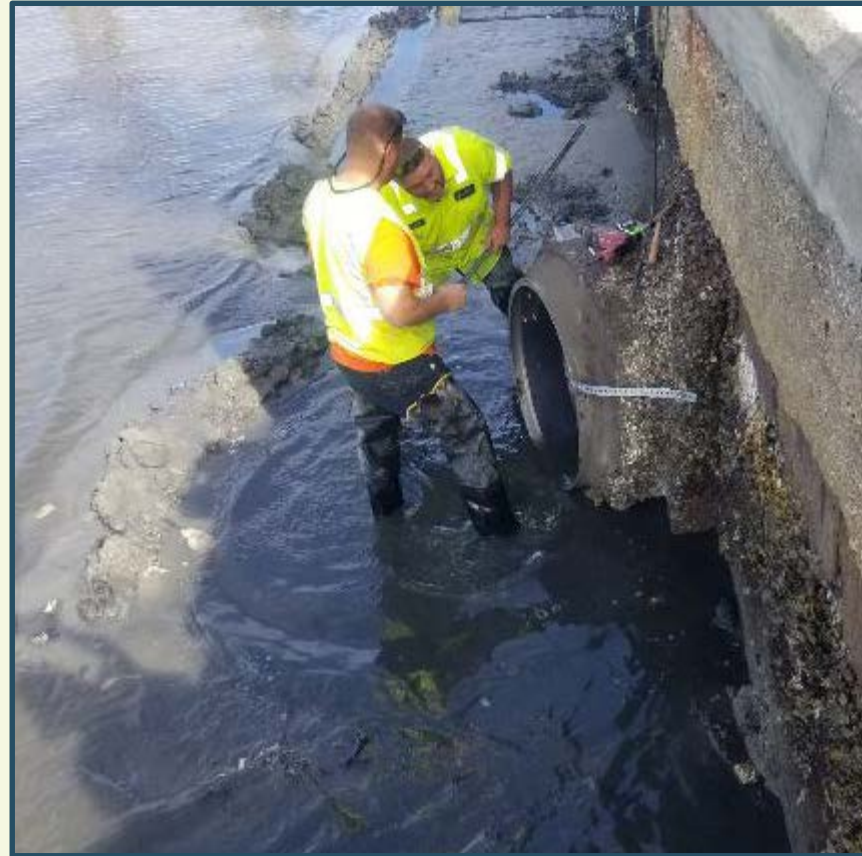
OF-0142 (After): Crew securing valve with straps onto outfall pipe
