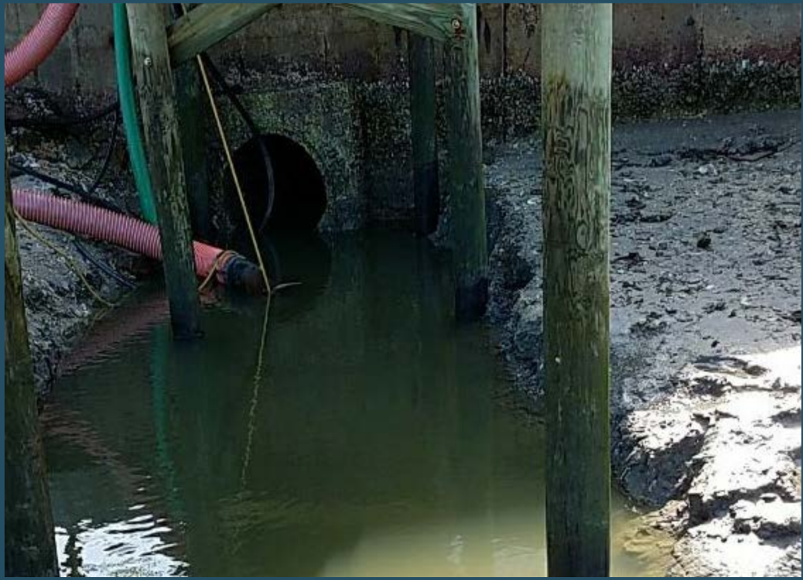
OF-0141 (After): Removal of silt at end of discharge pipe
