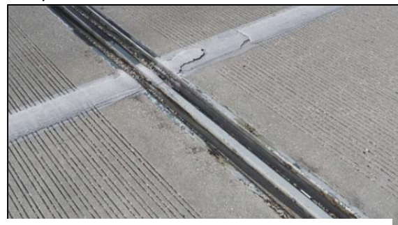
Figure 4.20: Expansion joints make for a rough crossing onto the Usina Bridge.
