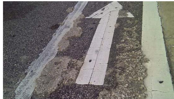
Figure 4.9: Accumulated concrete makes for a rough surface in the bike lane at the intersection of SR 207 and S. Dixie Highway.
