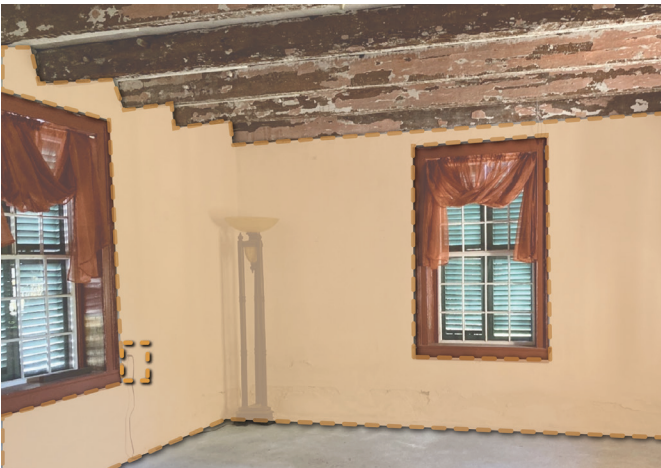
Replace inappropriate, non-permeable materials and finishes with historically appropriate materials and finishes like lime-based plaster that allow coquina walls to breathe and dry out after a flood event. Elevate electrical outlets.
