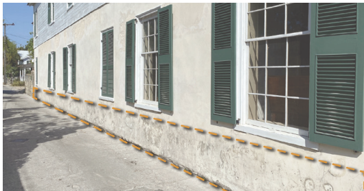
Rising damp appears as a darkened, stained area along the base of coquina buildings.
