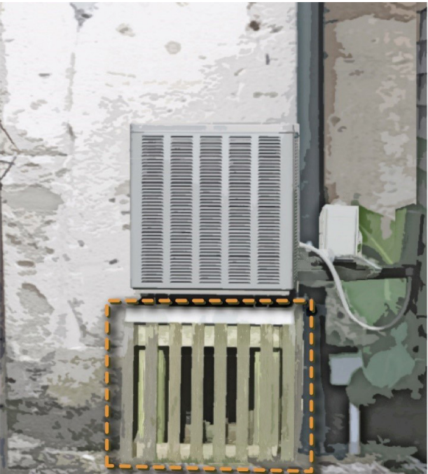
Elevate exterior equipment like air-handling units following the Historic Architecture Review Board (HARB) guidelines.
