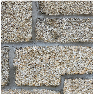
Dressed Coquina: units with two or more sides cut flat to be more geometric.
