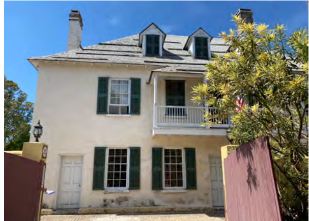
20 Aviles Street, St Augustine FL Hydraulic limewash finish on exterior
