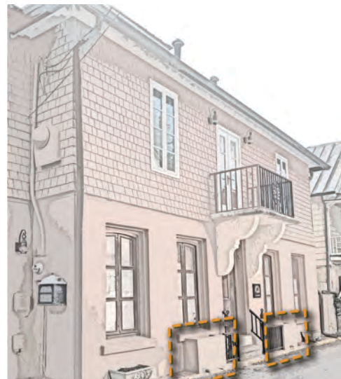
71 Marine Street, St Augustine FL Low Protective Walls at Crawl Spaces
