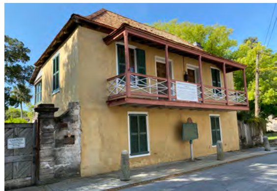
31 St Francis Street, St Augustine FL Vapor permeable finish on the exterior
