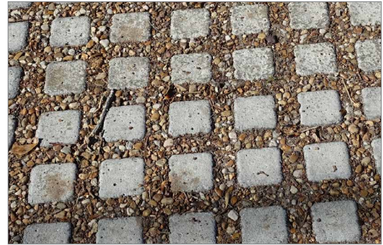
Gravel between driveway pavers is an attractive way to promote stormwater absorption and reduce runoff.
