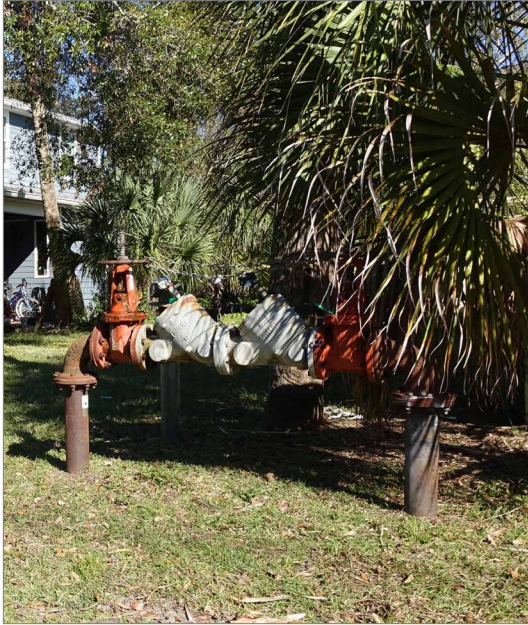
Municipal back flow preventers can protect contaminated water from entering the water supply in a neighborhood. Individual property owners can also install back flow preventers at water lines to protect their homes.
