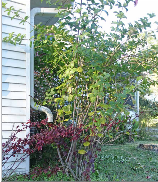
Downspouts should be oriented to discharge stormwater to allow flow away from and not towards building foundations.
