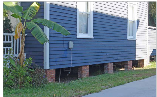
This open foundation house is supported by brick piers. Brick is a common pier material at historic homes. When elevating a house, brick can be applied over concrete to maintain the historic appearance.
