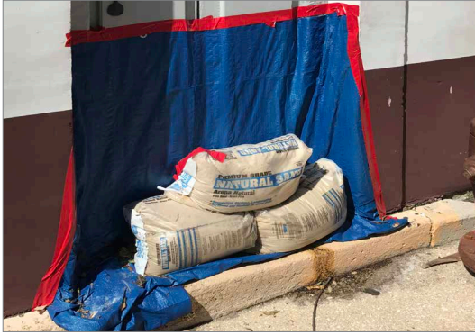
Sandbags are a mitigation measure that can reduce the impact of flooding. However, sandbags and associated plastic sheets must be properly installed to be effective. (Photograph courtesy of the City of St. Augustine.)
