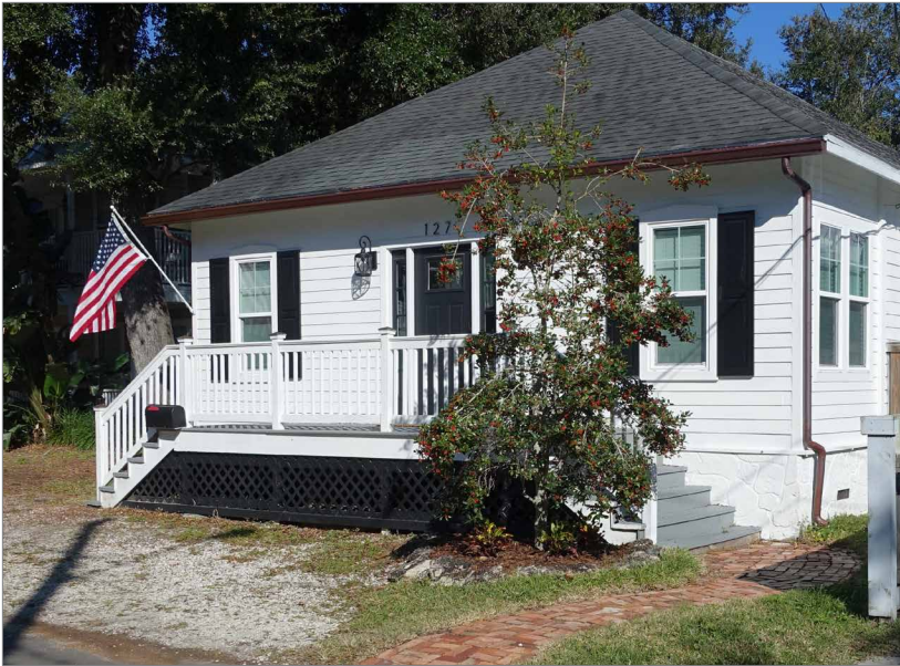
The porch is located approximately 3 1/2-feet above grade. The split stairs accommodate the stair length without discharging into the street.
