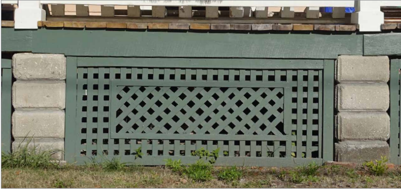
This custom lattice provides foundation screening between the piers. The use of diagonal or square lattice should be appropriate for the building's style.
