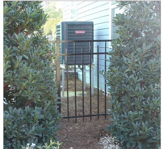
Exterior equipment should be installed so that it is elevated above the anticipated floodwater height. As the shrubs grow, they will provide visual screening.
