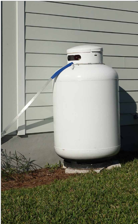
Propane tanks can provide an alternative fuel source however, they should be secured, such as the strap tie-down in this example, to prevent floatation during a flood event.
