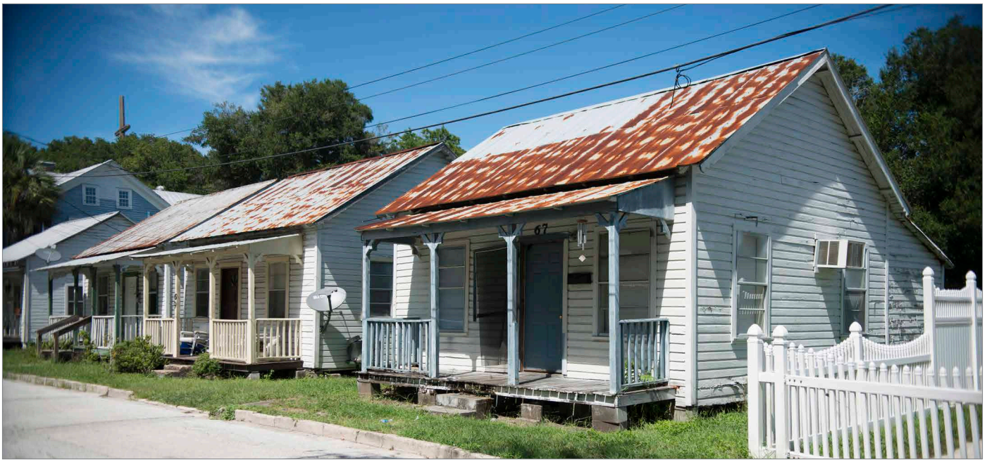
Poorly maintained buildings are more susceptible to storm damage from floodwater and high winds due to wear and tear on roof, clapboards, and associated fasteners.
