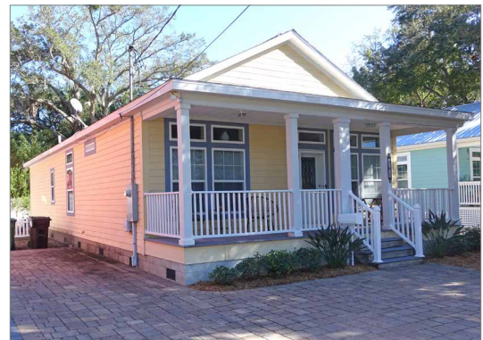
This home has a closed foundation with regularly-spaced flood openings along the side elevation.
