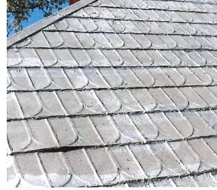
Stamped metal shingle roof
