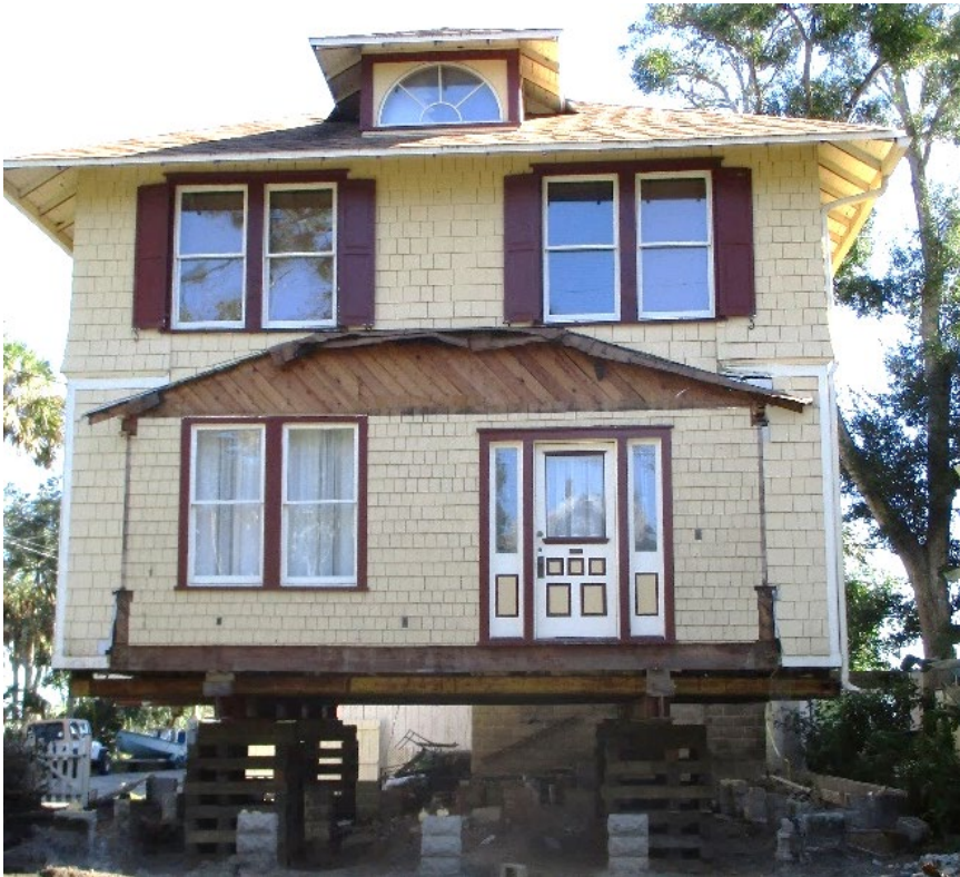
Foundation (and porch) was removed to allow for the building to be elevated to a new floor height for a flood mitigation project.
