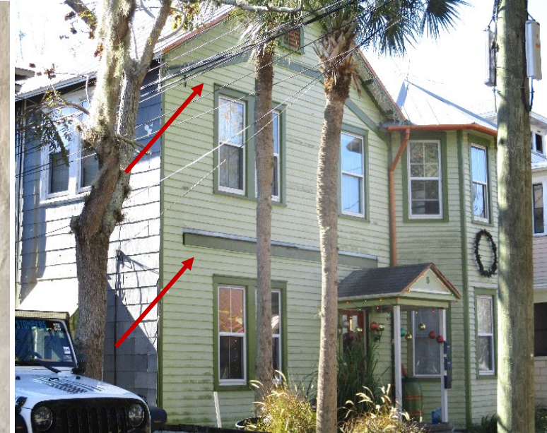
Evidence on the Sanborn map (left) and the building shows there used to be a historic two-story frame porch likely removed ca. 1930-1950s when asbestos siding was added. Reconstructing a compatible porch could be approved by staff.
