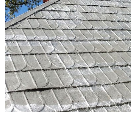
Stamped metal shingle roof
