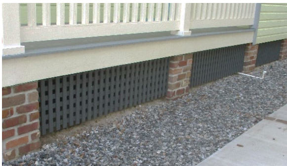
A new brick pier foundation matches historic materials and scale, as seen above
