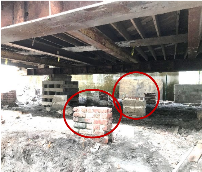
A building elevation project revealed unique coquina stone piers (background) along with traditional brick piers (foreground)
