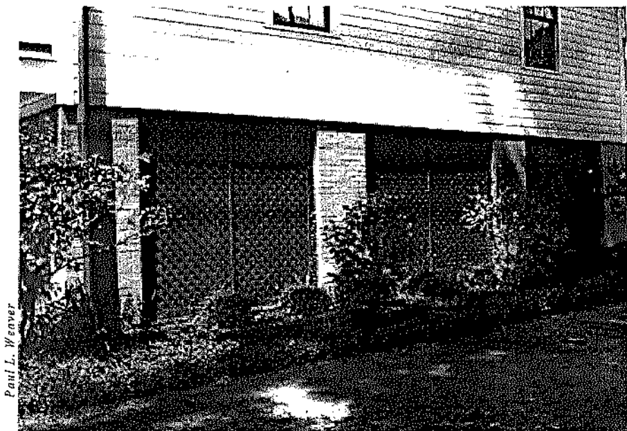
Lattice infill between brick piers.
