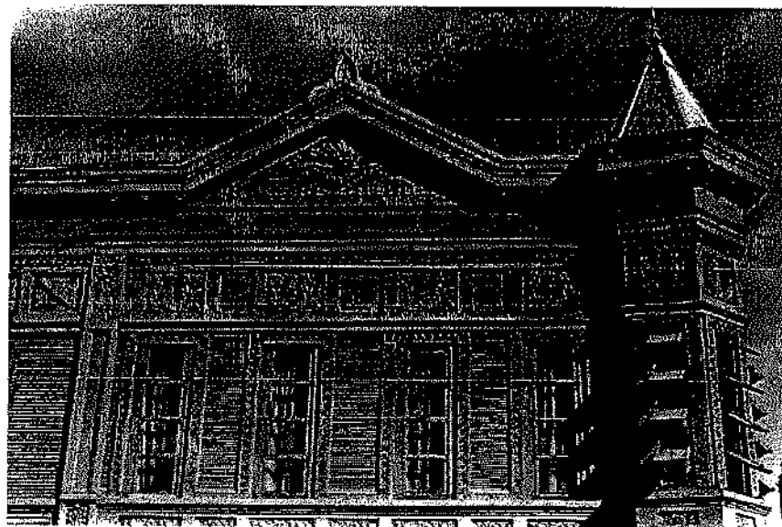
Pressed metal exterior cladding, Rogers Building, Orlando.
