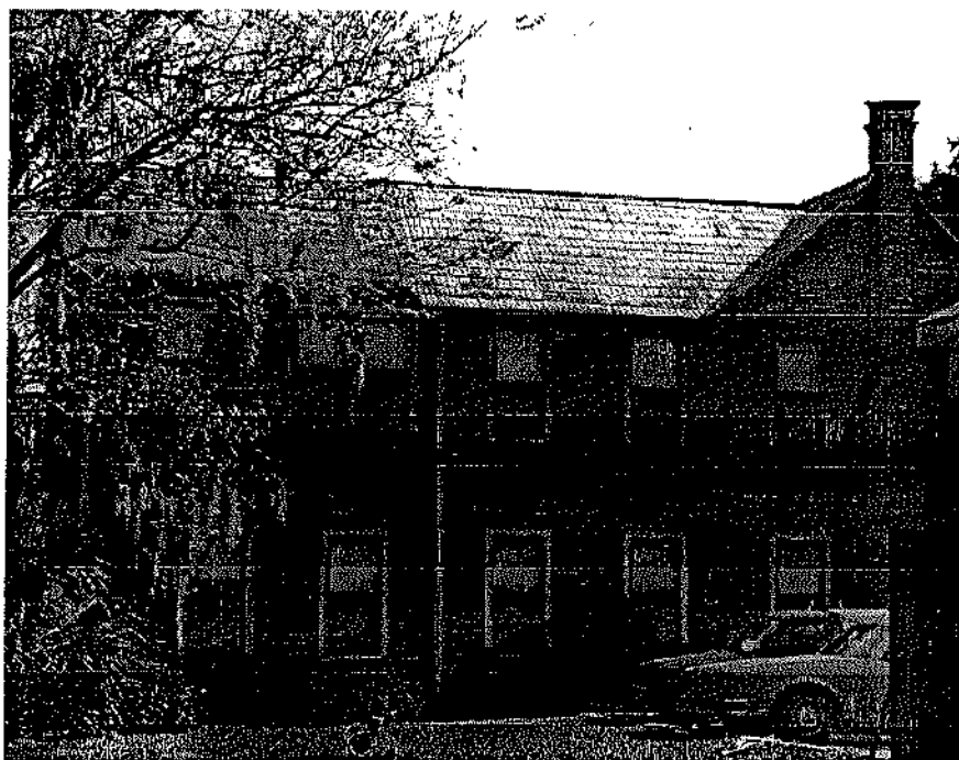
Metal, Gothic shingle roof, Bunnell, Flagler County.
