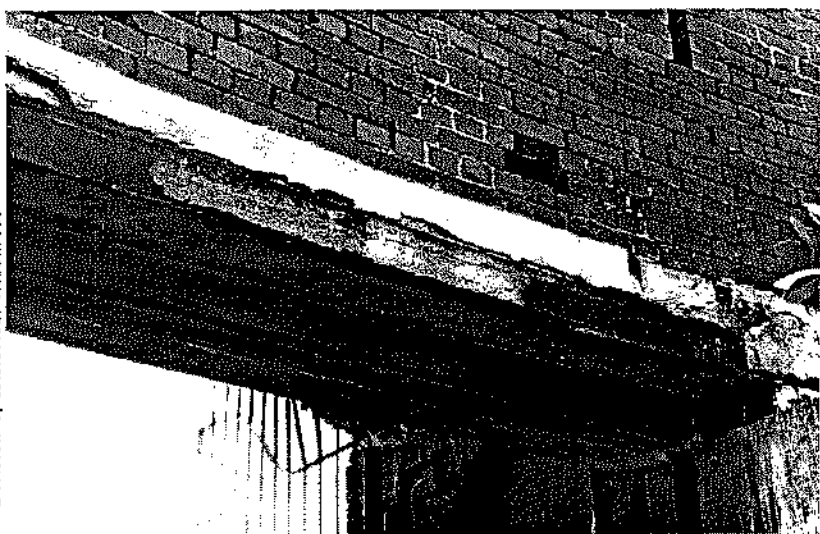
This brick wall requires repointing of mortar joints and replacement of missing features.
