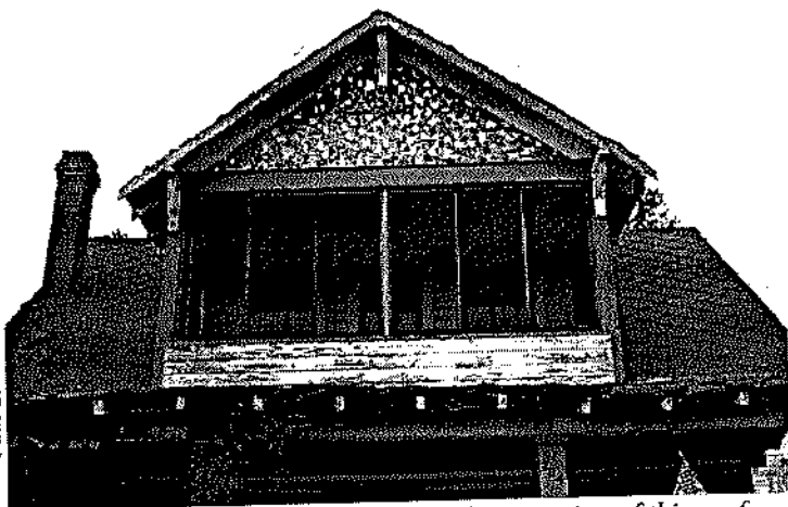
Deferred maintenance has resulted in deterioration of this roof.
