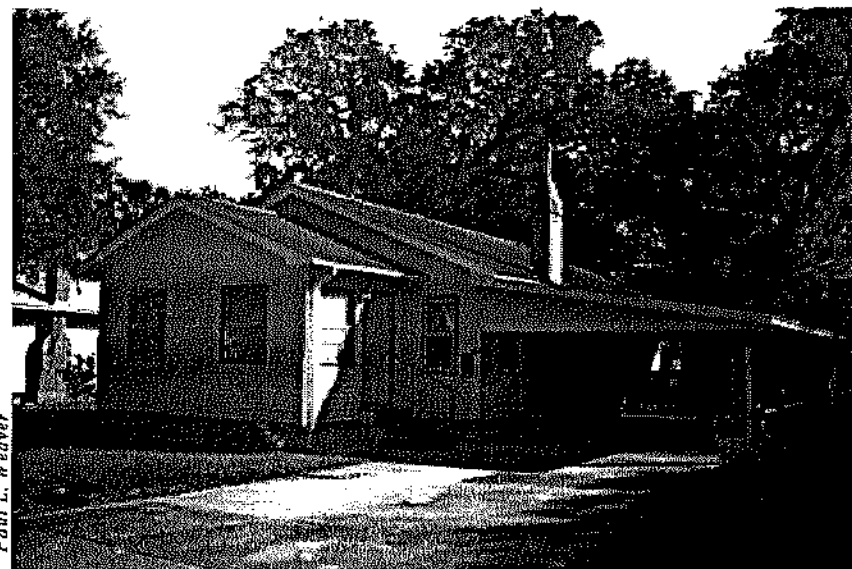
Vinyl siding has resulted in the loss of window and door trim and other wooden features.
