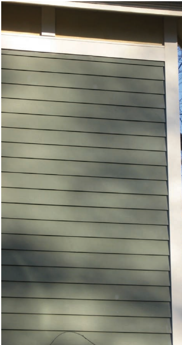
Cementitious siding was used to replace the deteriorated siding on this ca. 1869 dwelling in Fayetteville, Arkansas.
