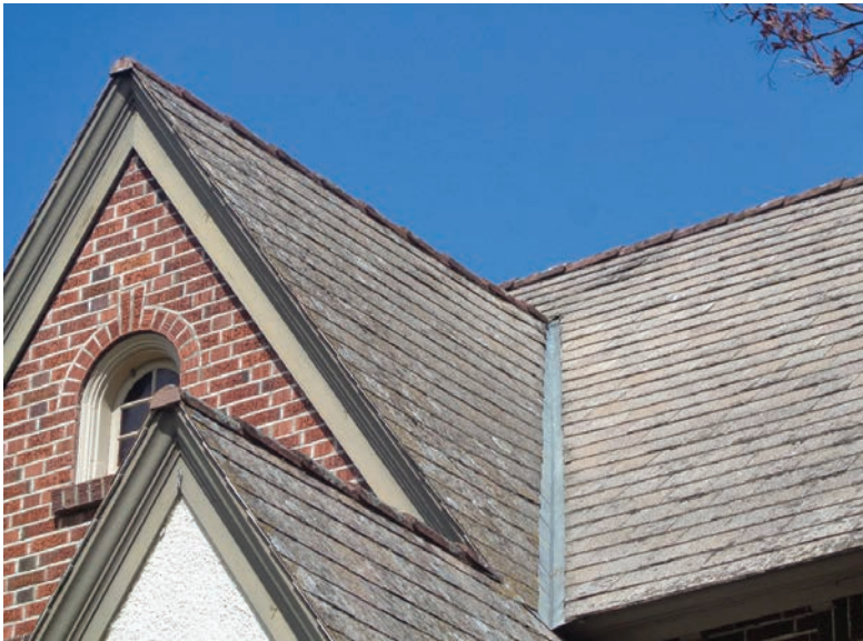
Numerous roof ridges with asbestos ridge tiles.
