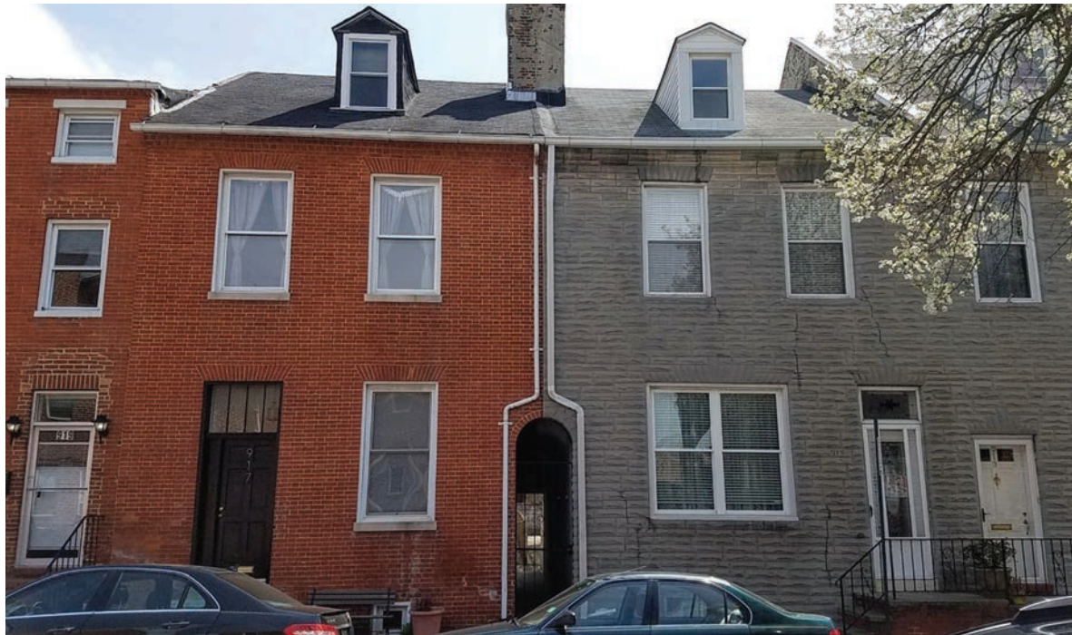
A contrasting double house with the original brick on the left and Formstone on the right on Stiles Street in Little Italy.
