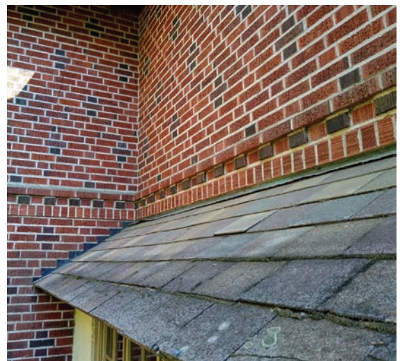
Closeup of roof tiles indicating thinness of the tile.
