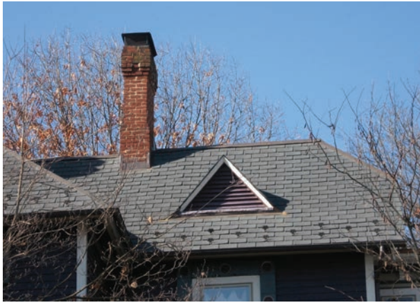
Example of an approved synthetic slate roof in Roanoke, Virginia.
