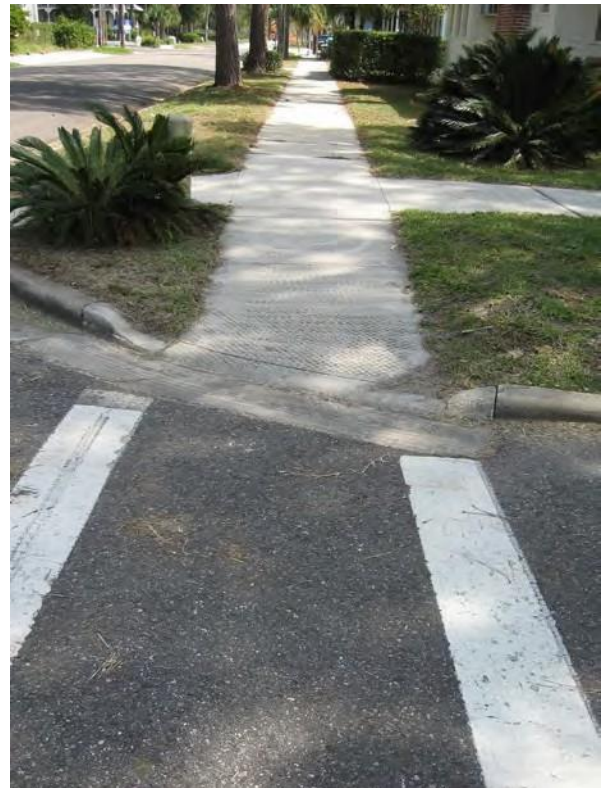
ADA curbing installed at South Eight and Beech Streets. Below: ADA curbing at South Seventh Street.
