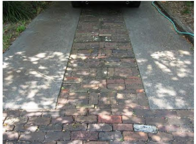
Driveways, like sidewalks, are often concrete. The "ribbon" design is a common historic design. The example at 119 South Seventh Street has brick infill, but often the ground surface is left natural.
