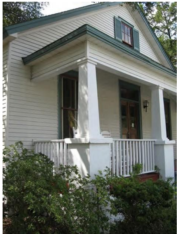
Porches on Bungalows such as this one at 406 Ash Street often have tapered wood posts on masonry piers.
