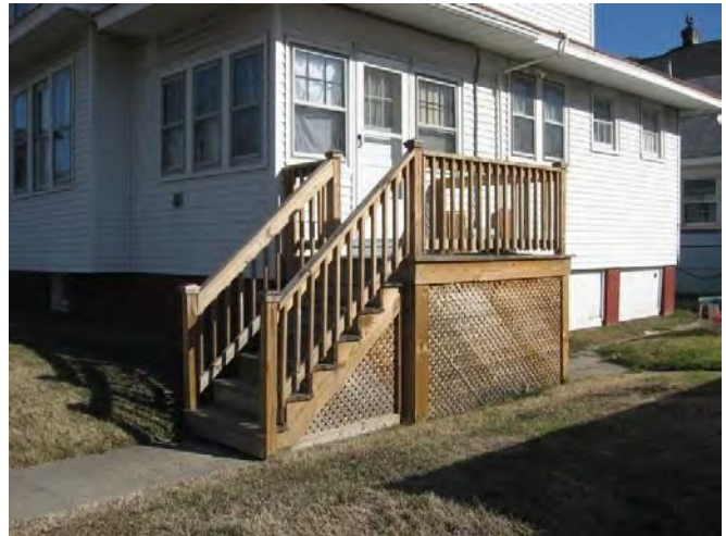
Rear decks should be simple in design with square balusters.
