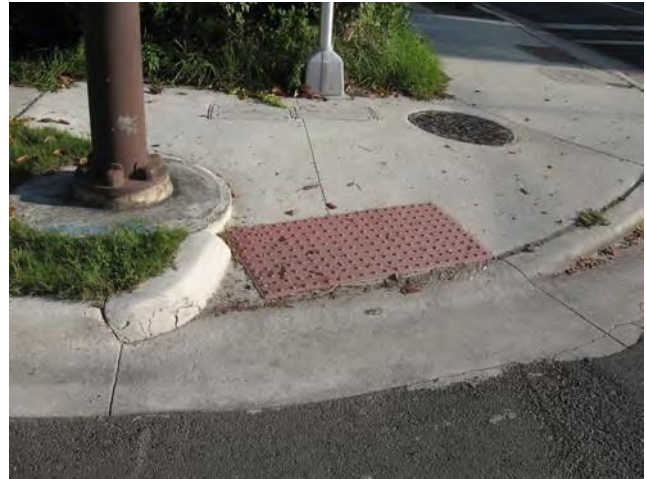
ADA curbing installed at South Eight and Beech Streets. Below: ADA curbing at South Seventh Street.
