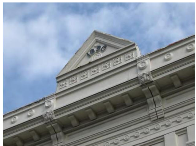
Retain and maintain historic roof elements such as the sheet metal cornice at 313-319 Centre Street, which is a character-defining feature.
