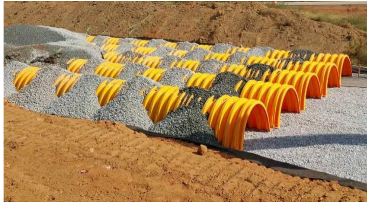
Figure 4.14 Underground Storm Water Detention System (Hydrology Studio 2020)
