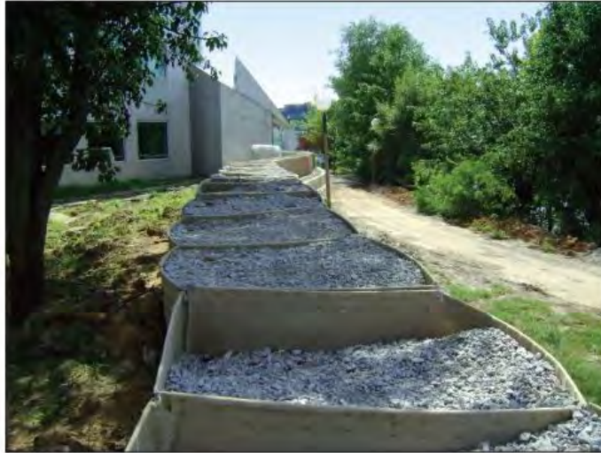
Figure 4.16 Gravel Filled Containers that Form a Flood Barrier (FEMA 2013)
