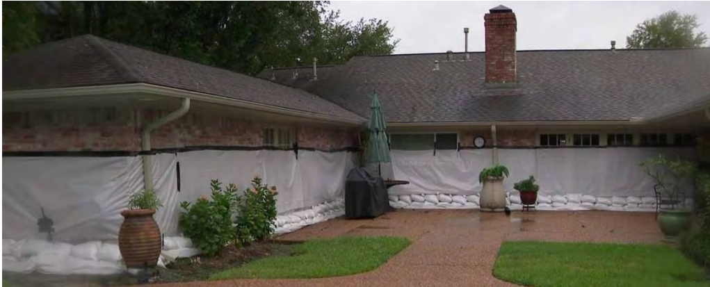
Figure 4.6 Temporary Plastic Sheetting Installation (Aragon 2017)
