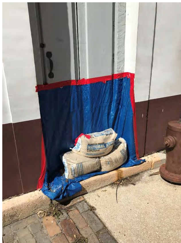
Figure 4.5 Homemade Temporary Flood Wrap Deployed in St. Augustine
