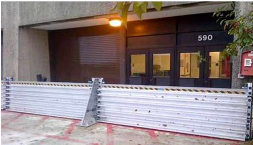
Figure 4.7 U.S. Naval Academy Temporary Stop Logs
