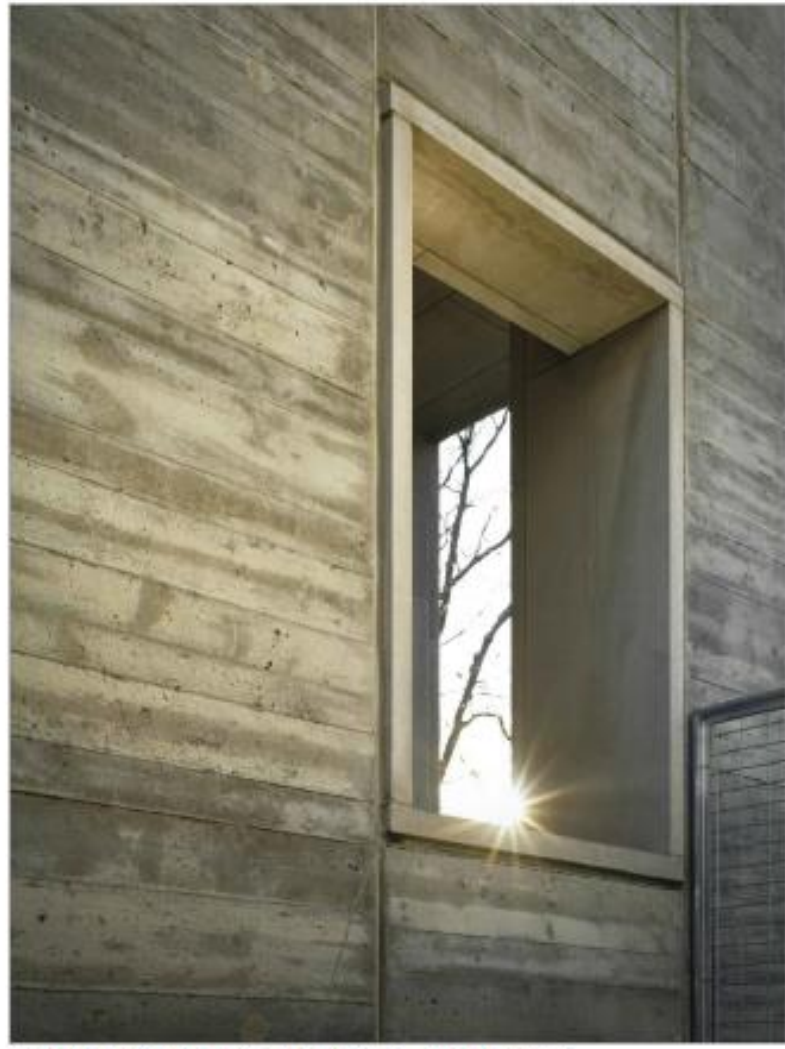
BOARD FORM CONCRETE WALL w/WINDOW
