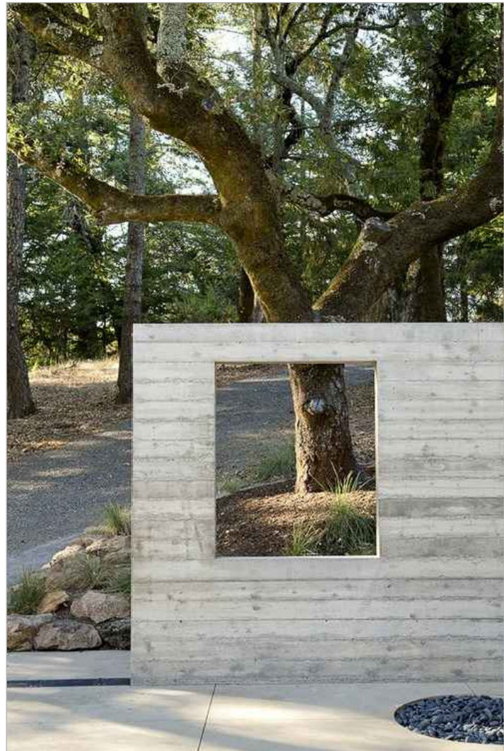
BOARD FORM CONCRETE WALL w/WINDOW
