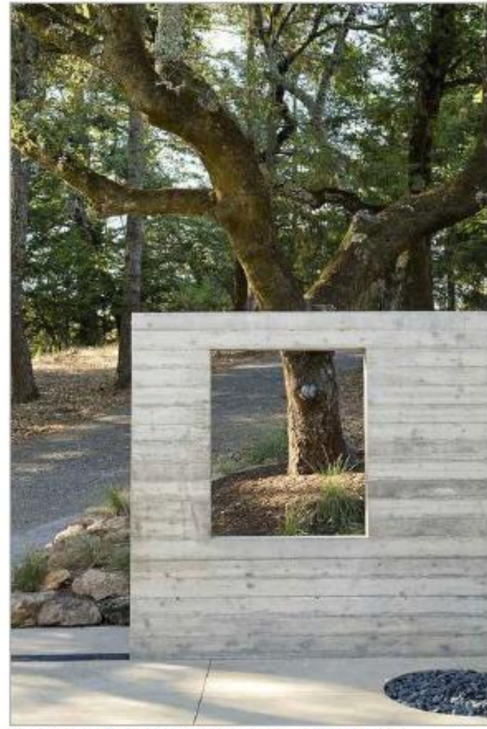
BOARD FORM CONCRETE WALL w/WINDOW
