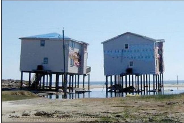
*Differential settlement of buildings thought to be a result of inadequate foundation embedment coupled with erosion, scour, and/or soil liquefaction (Surfside Beach, TX, Hurricane Ike).*
